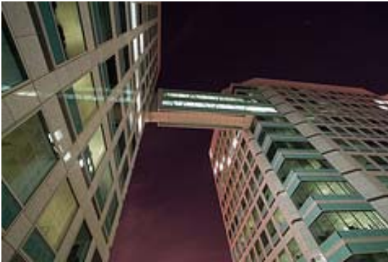
ADOBE Buildings San Jose, CA
